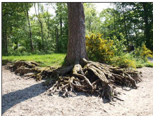
Exposure of tree roots at foreshore
