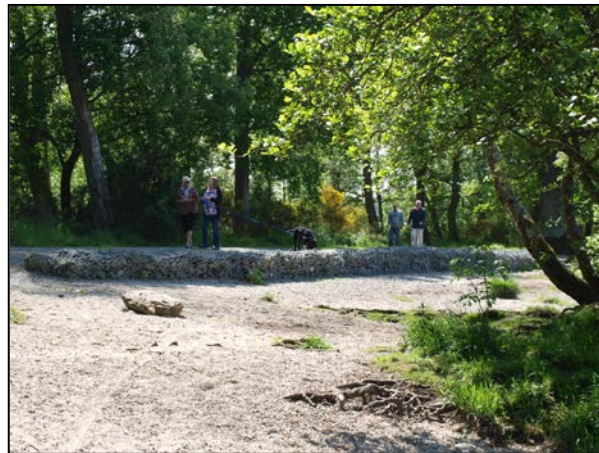
Revetment work along edge of loch shore path
