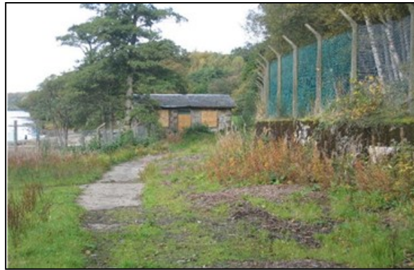
Boat House Prior to Restoration (West Dunbartonshire Council)
